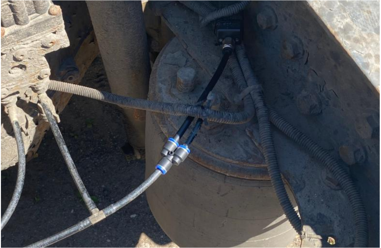
fig. 3.4. Connection of pneumatic line finished
