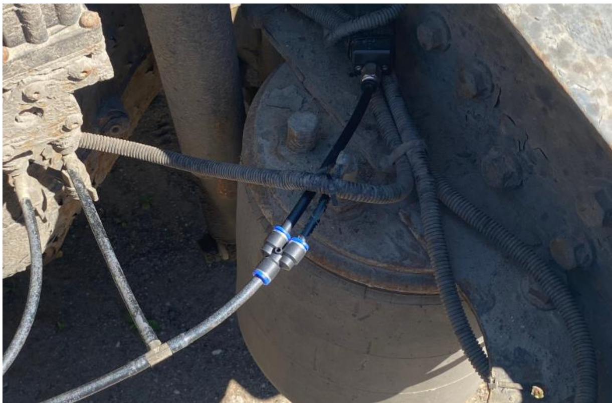
fig. 3.4. Connection of pneumatic line finished
